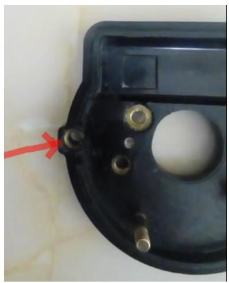
The brass washer indicated by the arrow is the return earth pick up point, this in turn is laminated via the Bakelite base plate to supply a earth return to the Condenser and C/B points.
