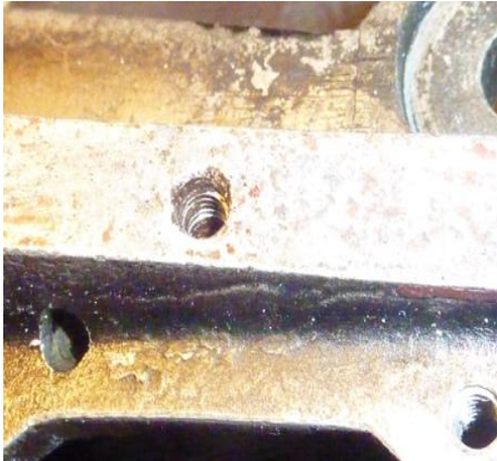
Typical of many sunken 'Helicoils'
